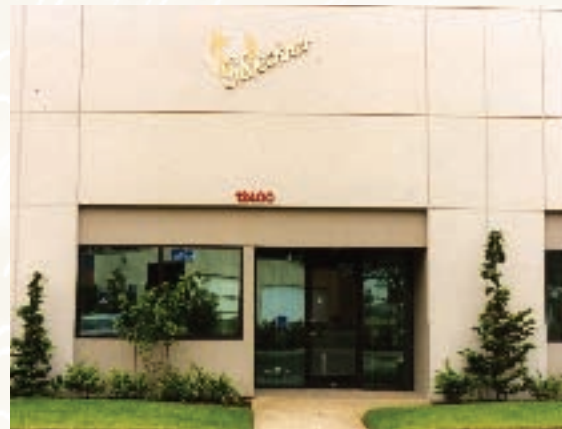
West Coast Office & Bulb Storage Facility Clackamas, Oregon
